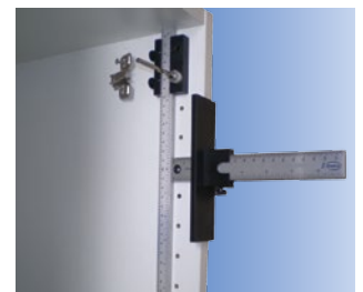
Drilling for placing invisible hinges.
