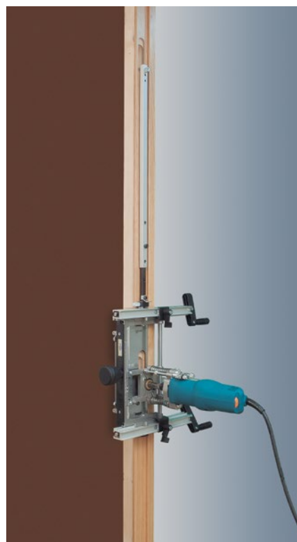
Making the second recess on the frame.
