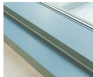
Working with composite panels (Alucobond® and similar) using routing and folding method.
